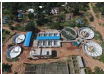
Water Treatment Plant at Dar es salaam
